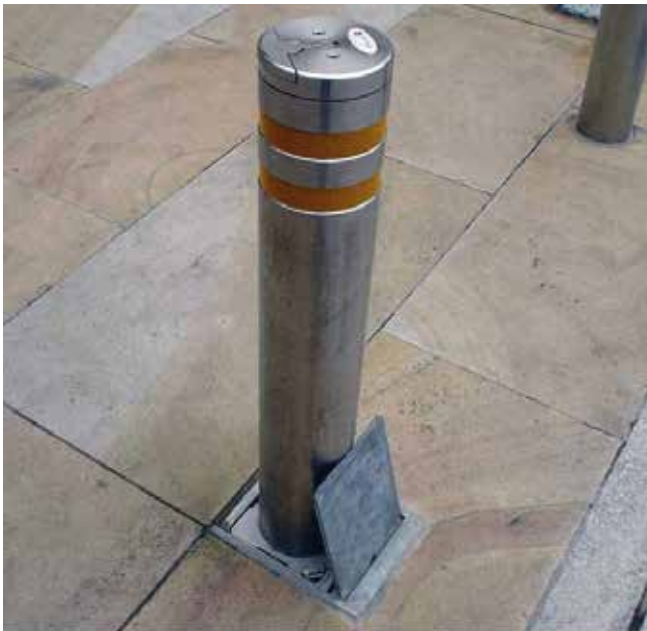
Image 8. Manually controlled bollard.
