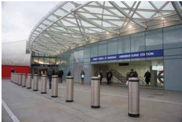
Image 5. Fixed bollards installed at a London underground station.
