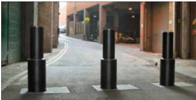
Image 7. Shallow-mounted automatic bollards.
