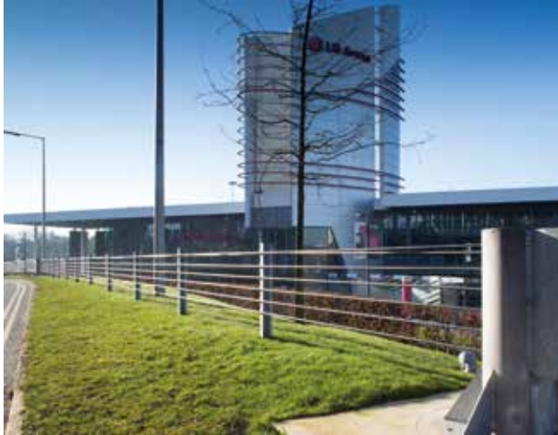
Image 11. Bristorm wire fencing.
